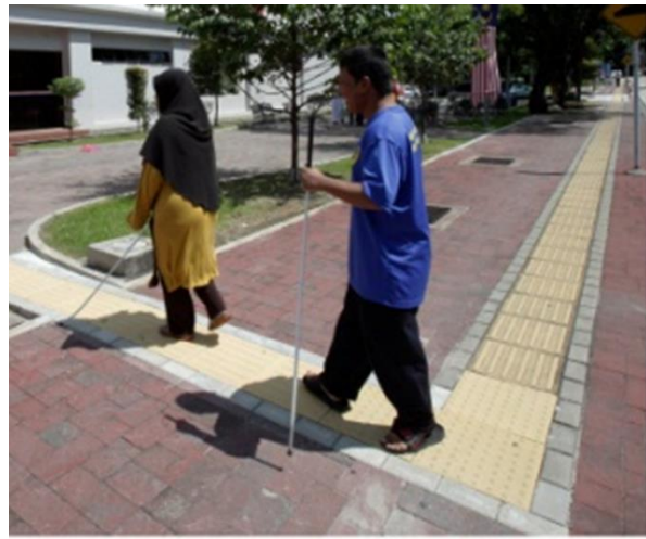
Figure 29: Walkways for person with disability
