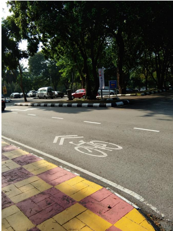
Figure 39: Installation of shared lane road markings (sharrow) in early 2018 along Lingkungan Budi route
