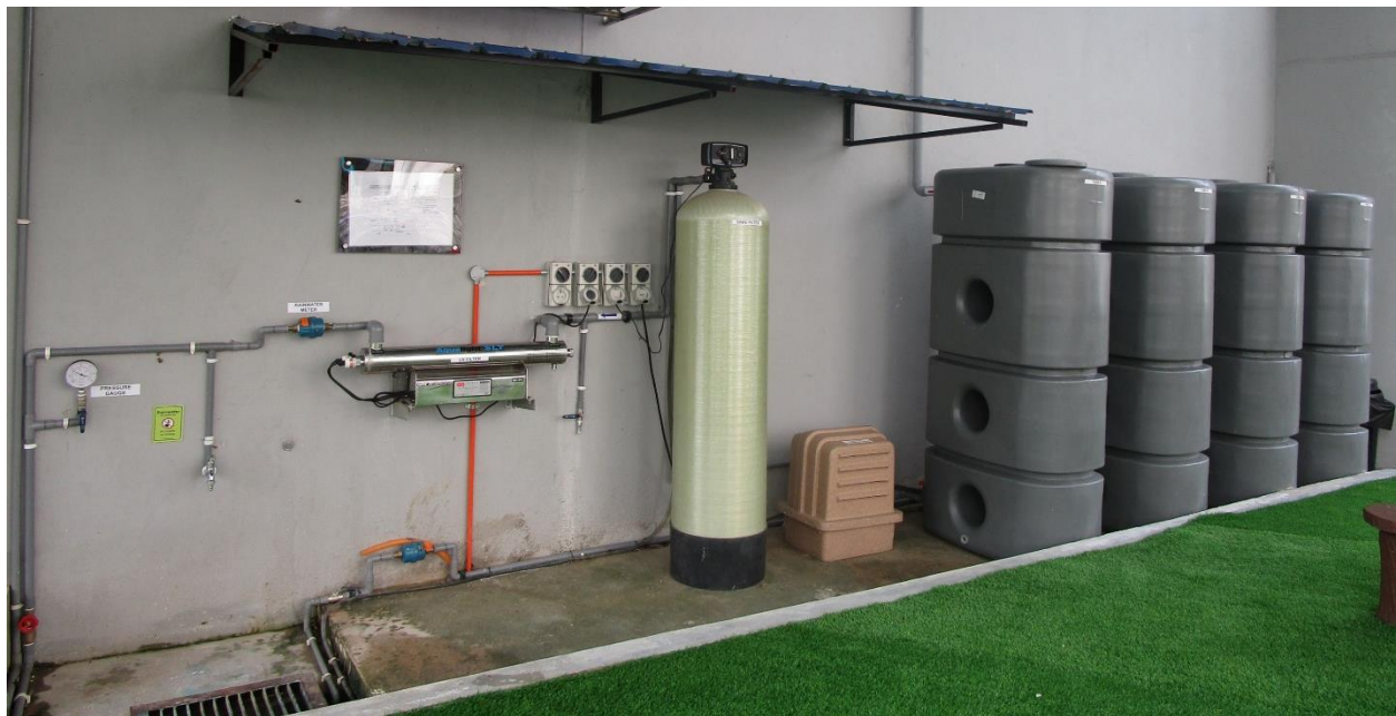
Rain Water Harvesting System
