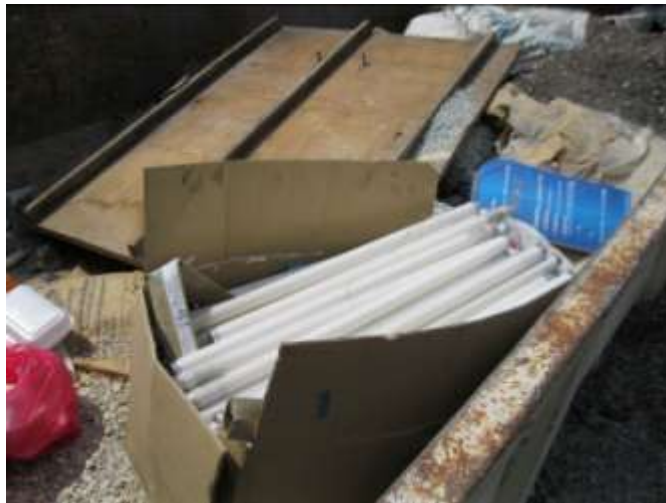
Figure 3.4: Fluorescent lamps found in open top bin for renovation waste
