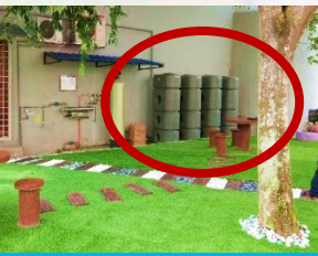
Installation of 'Mr. Thimble' and Rainwater Harvesting System at Surau in campus to reduce water consumption
