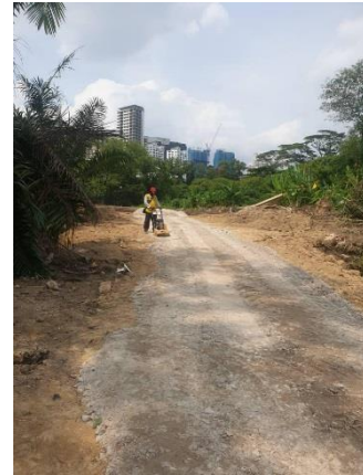
19 July 2019 Adding gravel stone layer as the base foundation
